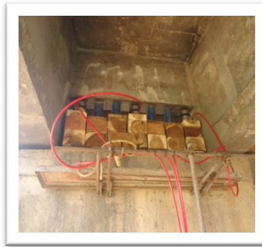
Figure 5: Cross Girder Lifting in Progress
