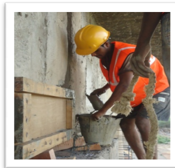
Figure 6: Micro Concreting at the Bearing Region of Main Girder
